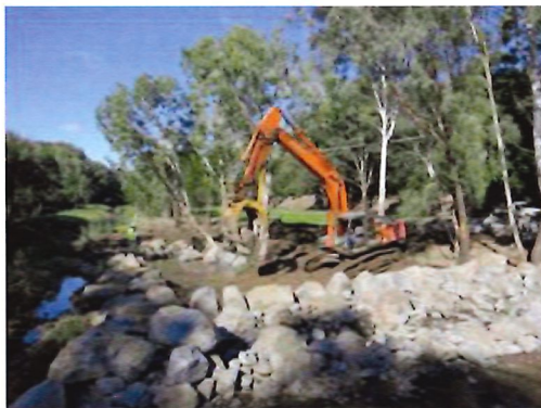
Figure 8: The excavator uses the 'grab' to place the boulders (up to 4 tonne each) into place while the Queensland Fisheries staff check levels and 'V' channels to create eddies and easy migration paths for fish.
