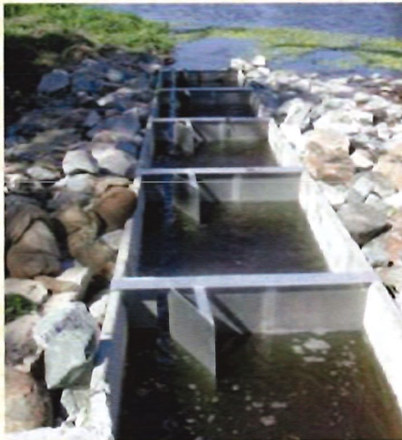
Vertical-Slot Fishway, Gooseponds Creek, Mackay City management area (Photo by Tim Marsden)
