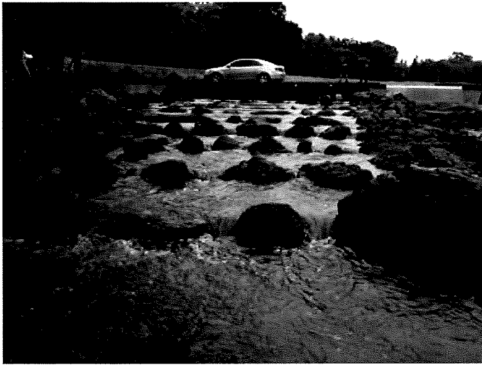
Figure 10: The fully functioning fishway! What a beautiful sight.
